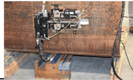
Crawler to Delivery Camera Systems within Refractory Air Slots
