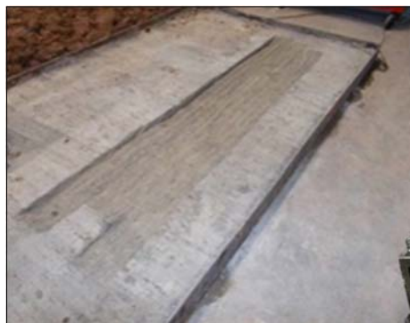
3 Passes on 7:1 Mix Concrete
