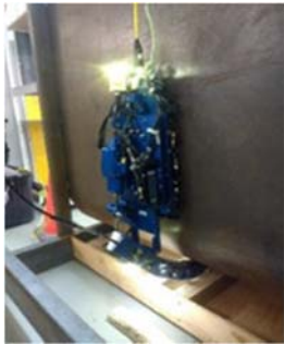
Primary Tank Bottom Inspection Crawler
