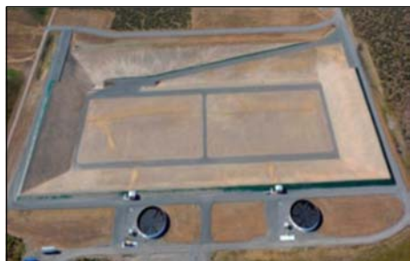
Integrated Disposal Facility
